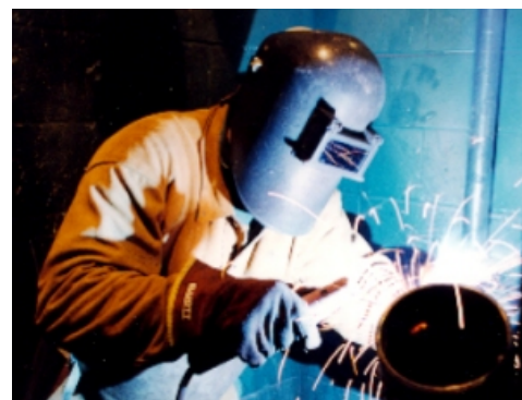
Figure 3.3.c. Welding produces fumes. As the metal melts, and the welding rod and flux covering is burned, fumes are produced. These fumes can cause irritation to the nose and lungs.
