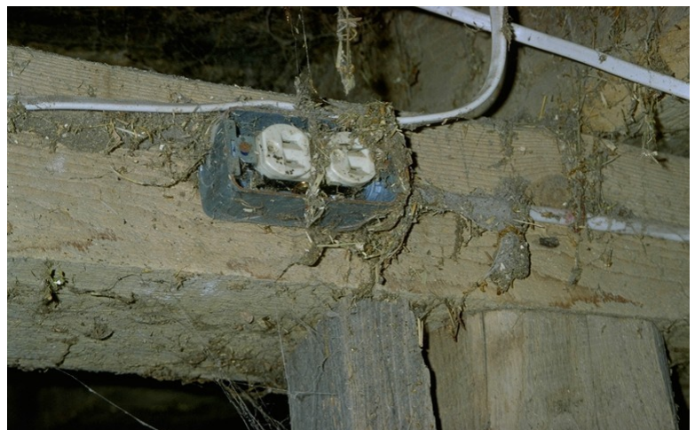
Figure 3.7.c. Dusty, dirty conditions in agriculture contribute to increased fire hazards. What materials in this picture are considered Class A fuel sources?
