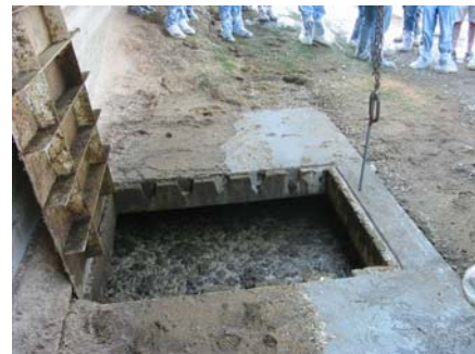
Figure 3.11.a. Manure storage pits are often found below ground level. They are covered until time to pump them out. The agitation and pumping releases toxic gases.
