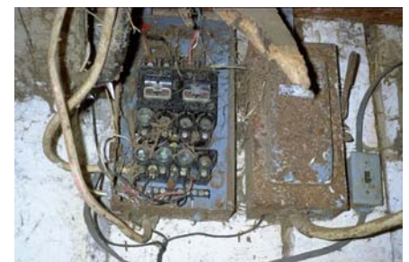
Figure 3.6.d. Improper electrical wiring methods and materials placed into a hostile farm environment can lead to fires and electrocution of people and livestock.
