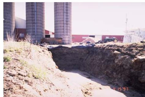
Figure 3.8.c. Trenches and pits in agriculture pose risk of sidewall cave-in and entrapment of the worker. Death by crushing can result. Suffocation can also occur.
