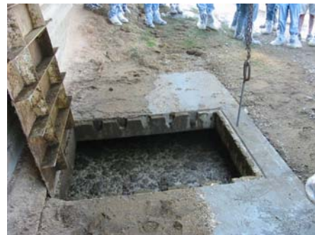
Figure 3.8.a. A manure pit is a confined space work area. Many lives have been lost in manure pits due to toxic gases and lack of oxygen.
