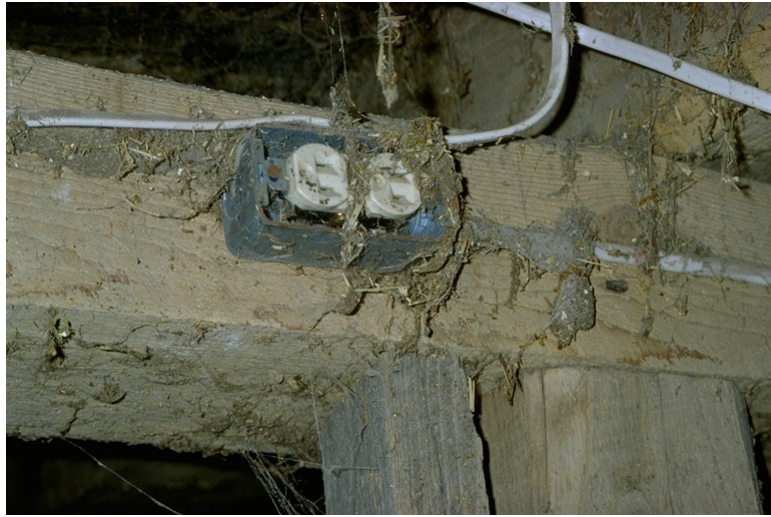
Figure 2.6.b. Fine particles of dusty materials burn quickly. A spark or overheated wire can ignite the fine particles with the resulting fire causing thousands of dollars of damage. What problems can you identify in this picture?
